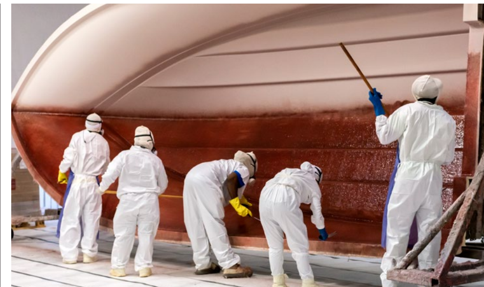
THE SPRAY'S THE WAY Each application of resin and fiberglass contributes to the boat's overall strength, reliability and ride quality.
