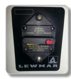
The windlass breaker is located in the head/console compartment.
